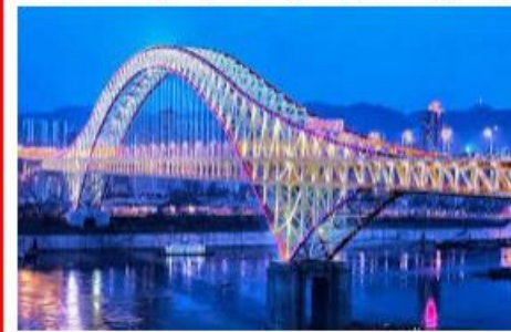
Chaotianmen Bridge (Chongqing, China) – world's longest arch bridge - Design institute of China Railway Major Bridge Engineering Group
